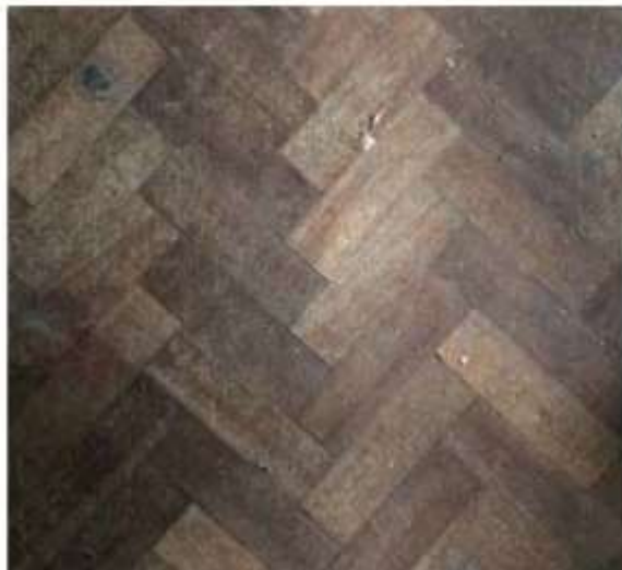
Herringbone timber floor
