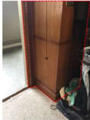
05 Existing timber wall lining 1:NTS
