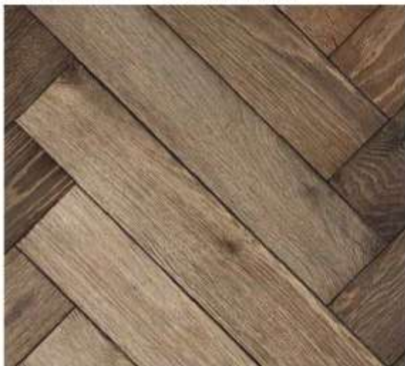
Herringbone timber floor
