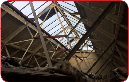
Existing asbestos and roof damage
