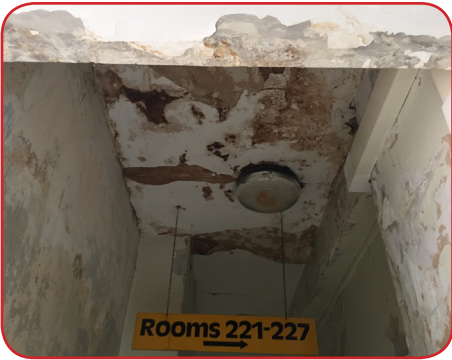
Roof damage, water ingress and deterioration of finishes
