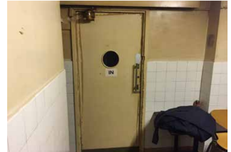
Item description: Internal timber doors with vision panels (multiple locations)
