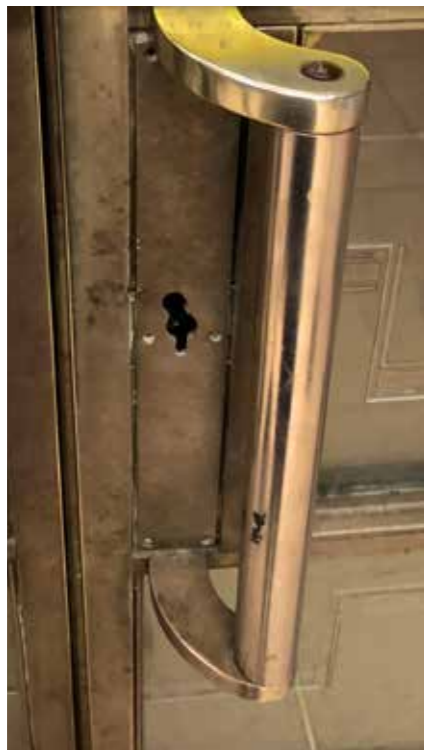
Photographs of original ironmongery to be salvaged and reused
