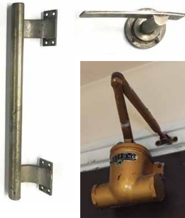
Photographs of original ironmongery to be salvaged and reused
