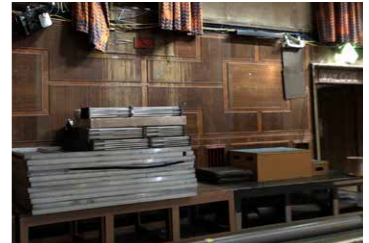
Item description: Timber panelling in the Assembly Hall (example of panelling that can be rejuvenated and reused in its totality)
