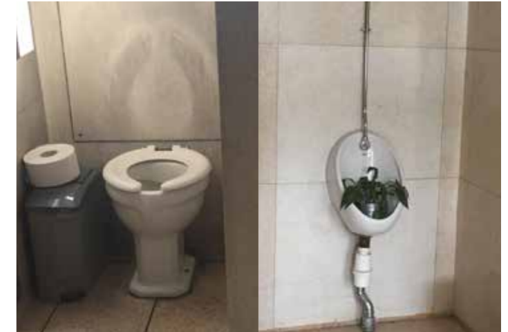
Item description: Original WC pans and urinals
