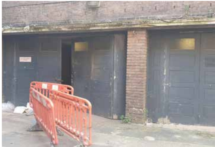
Item description: External garage doors (LG.22, LG.22a, LG.22b)
