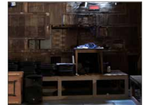
04 Replace full panels NTS (including veneer, timber backing and framing)
