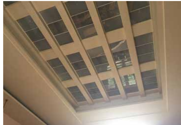
Item description: Laylights in the Council Chamber and Assembly Hall
