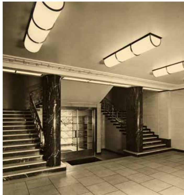
Photographs of original entrance doors from RIBA Archives
