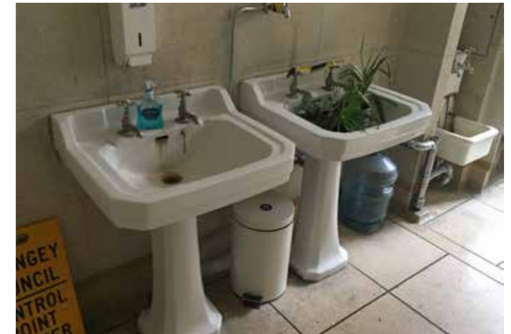
Item description: Original basins including cleaners' sinks
